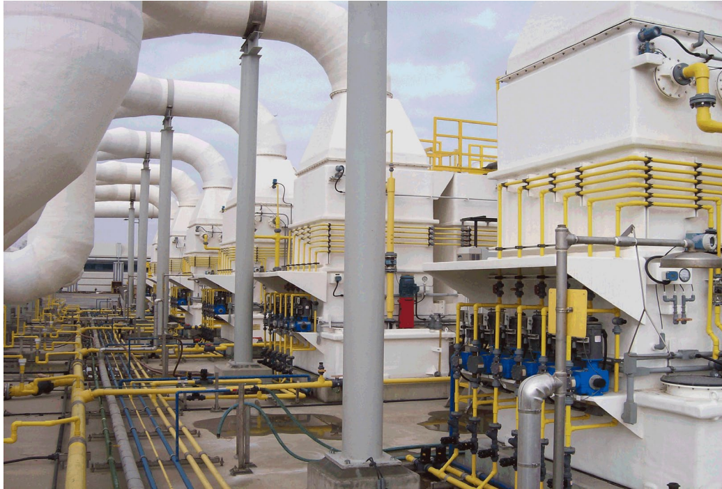
PRIMARY TREATMENT CENTRALIZED CHEMICAL SCRUBBERS
