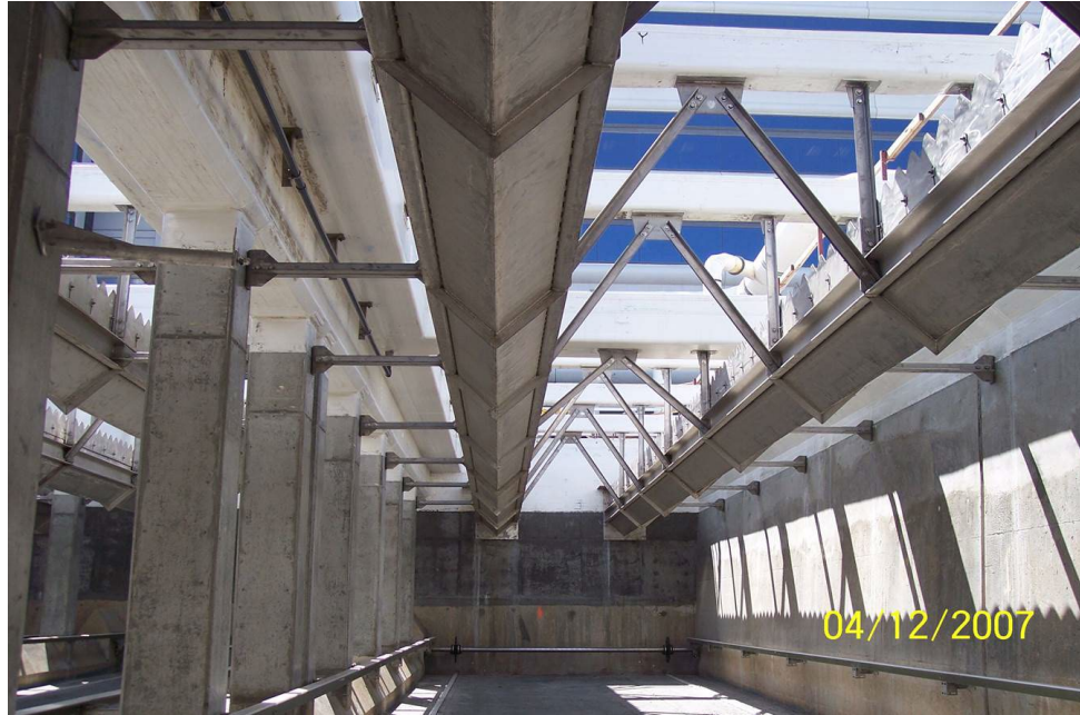
PRIMARY SEDIMENTATION TANK BAY
