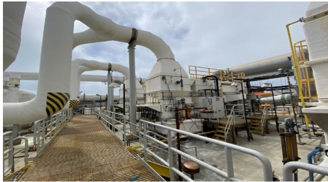
REFURBISH PRIMARY TREATMENT FOUL AIR SCRUBBERS
