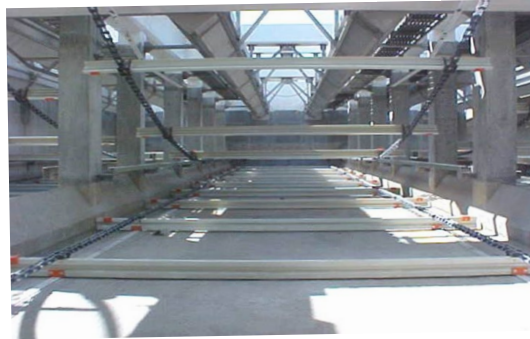
REPLACE SLUDGE HANDLING EQUIPMENT
