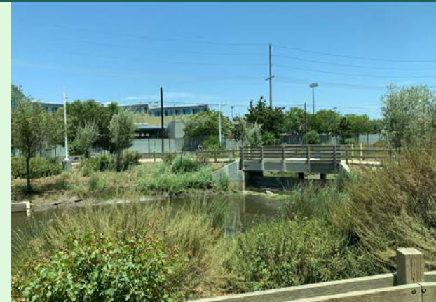
Pedestrian bridge over the wetlands.
