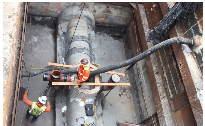
North Outfall Sewer Rehabilitation
